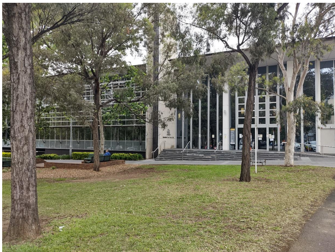
Photo 2: Bankstown Court House
