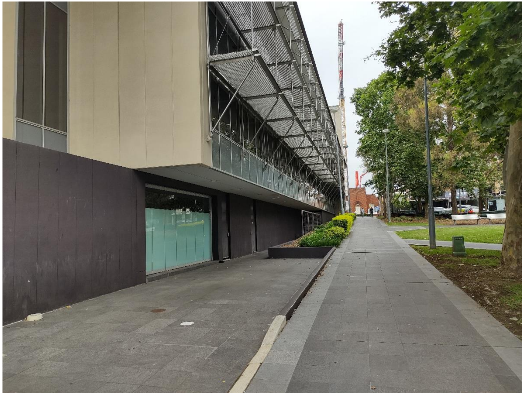
Photo 3: Bankstown Court House
